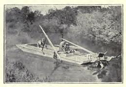
Fig. 101.—Motor Punt Weed-cutter. (Saunderson, Bedford.)
